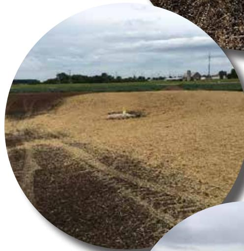
*WASCOB seeded down. Berm and tile inlet visible. Slopes graded to maintain productive cropland.*
